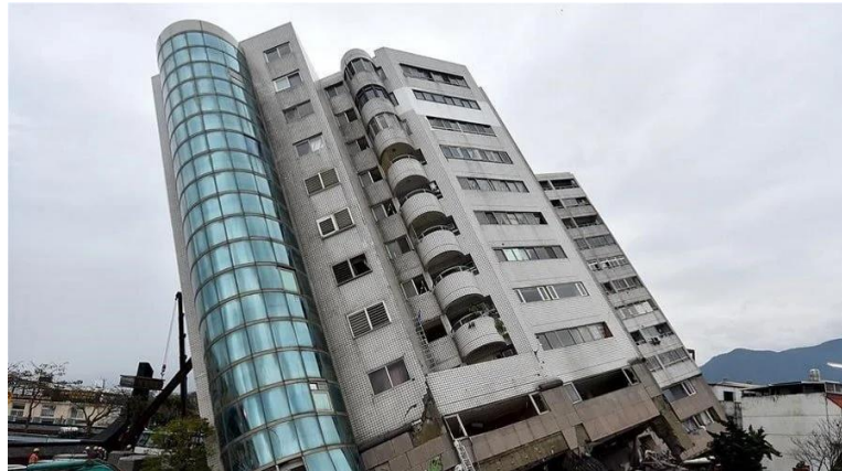
FIG. 1. EARTHQUAKE EFFECT ON TALL BUILDING[4].
